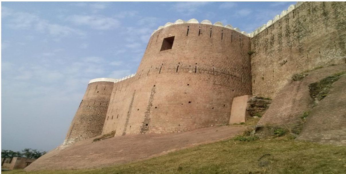
Figure 1.2: Bhimgarh Fort - Reasi (2014).
